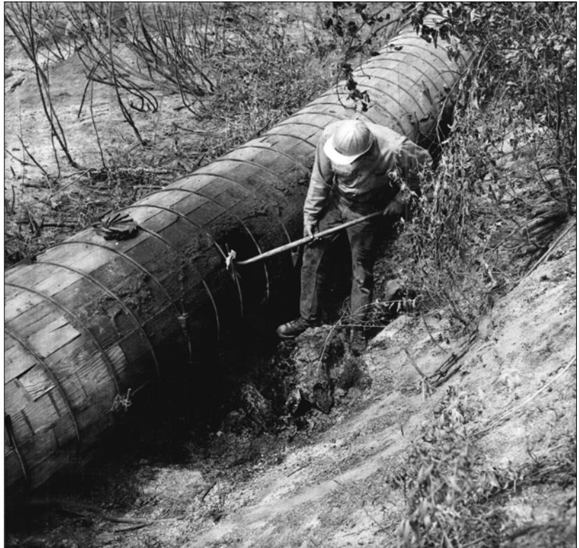
Besides wooden flumes, continuous wood stave pipes were used to collect and distribute the water used to irrigate the growing number of acres of orchards in the Manson area, which numbered 3,767 in 1929. These pipes continued in use until 1979. This photo was taken in 1970.
