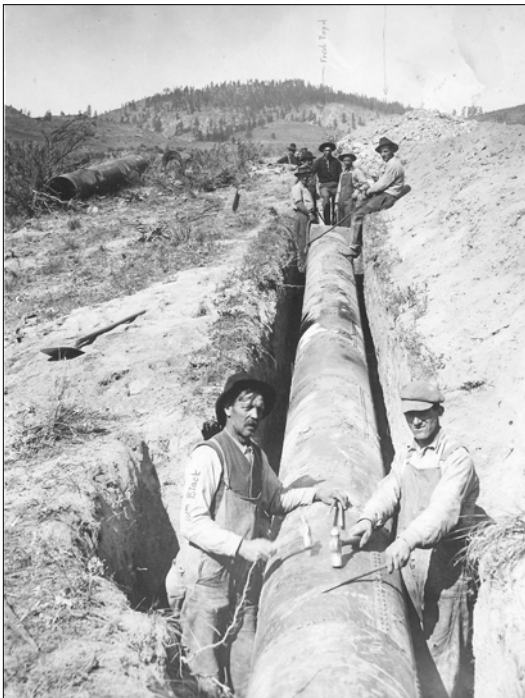
Manson siphon, 1910, below Antilon Lake; siphons were used to transfer water over a barrier, such as a canyon.
