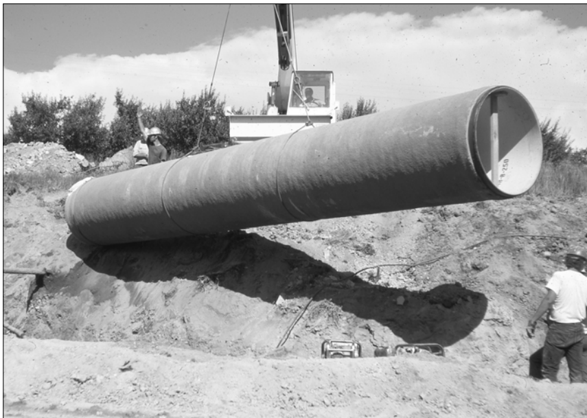
In 1972, installation of concrete-coated pipes was accomplished with a machine and a few men.
