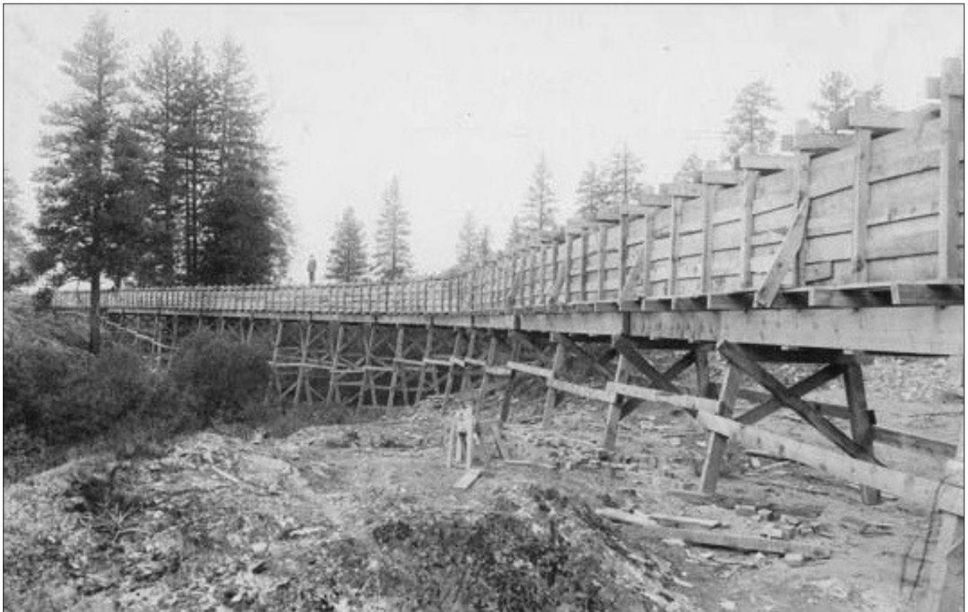
The flume to Antilon lake. The original photograph is captioned, "Supply Flume 14 miles long. Capacity 150 cu. ft. No timber in this flume comes in contact with the earth. All the posts stand on solid rock footings." By L.D. Lindsley, 1911.
